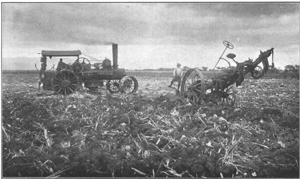
How the plowing is done. A stationery engine draws the big plow toward it by means of a wire cable.
