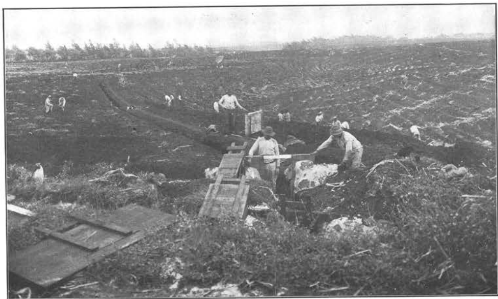
Where the land slopes the flumes are made to float the crop of cane to the sugar mill, perhaps miles distant.
