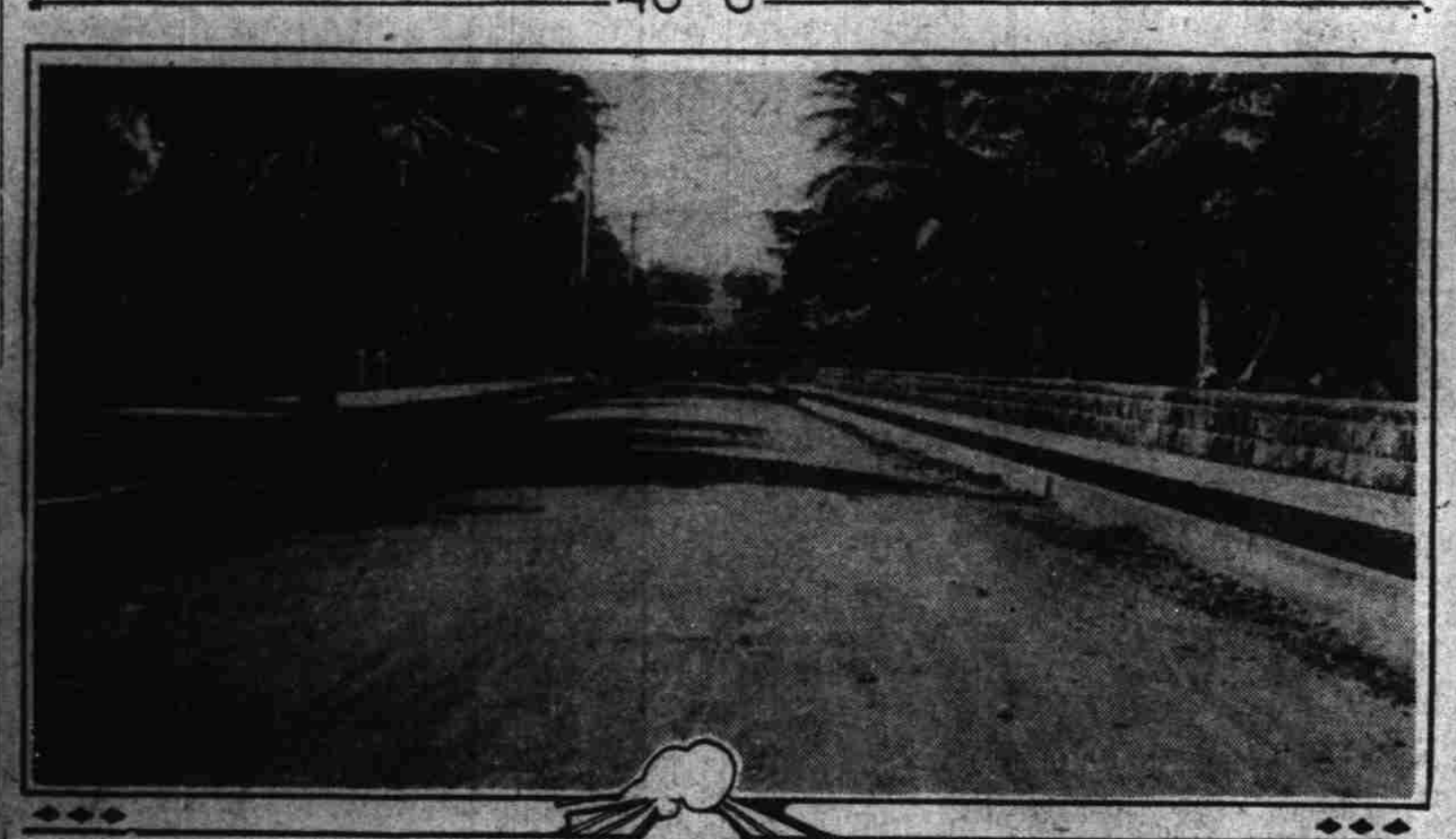
Pictures and sketch show how "sidewalk area" may be utilized for putting down public pipes and mains without tearing up street, the utilities going down in the earth strip. The lower photograph shows a completed Hilo street.
