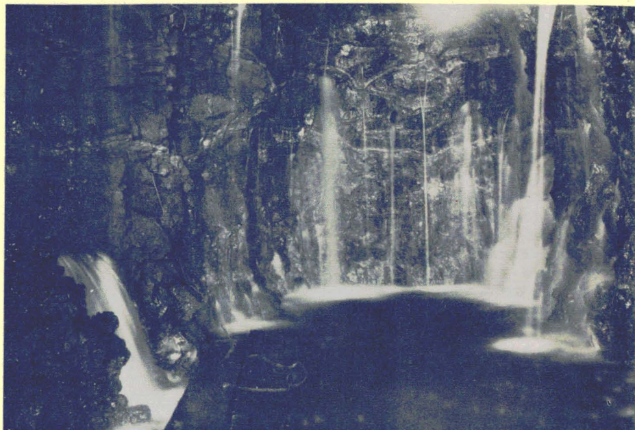
One of the newest types of water installations in Honolulu is the skimming tunnel. Above, water surges into the Halawa tunnel from the water-bearing rock below the surface of the fresh-water pool. Below, powerful pumps bring it to the surface.
