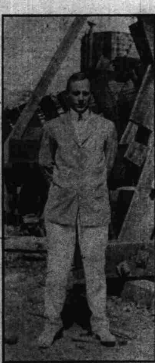
Civil Engineer E. R. Gayler
