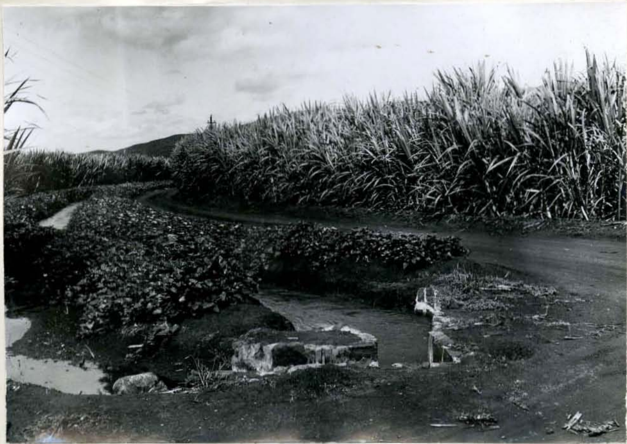
Figure 13 - Sugar cane in the apron area west of Kipapa Gulch at about 600 feet, showing a field road and parallel main contour ditch with diversion gates at a road intersection. Negative No. 21780.
