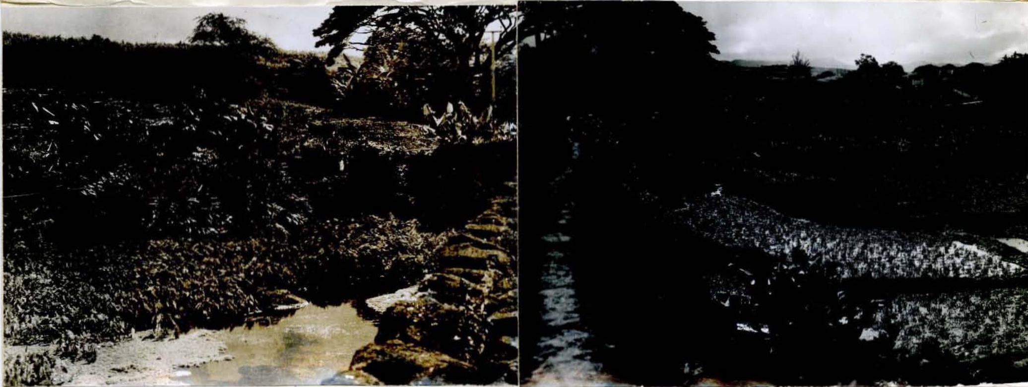
Figure 3 - View northeastward along wall to chief outflow point, Kalauao Spring. At left is the spring pool with water standing at about 13 or 14 feet above sea level. The outflow of water through a pipe is concealed in the near foreground on the right. Near and middle ground at the right consists of irrigated terraced gardens for taro and cress. Figure 4, following, is a view looking toward the camera position for this picture from a point near the apex of the wet gardens. Negatives No. 21620-21.
