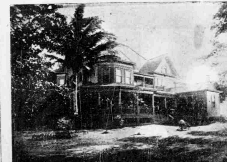
THE RESIDENCE OF MR. FRANK HUSTACE.
