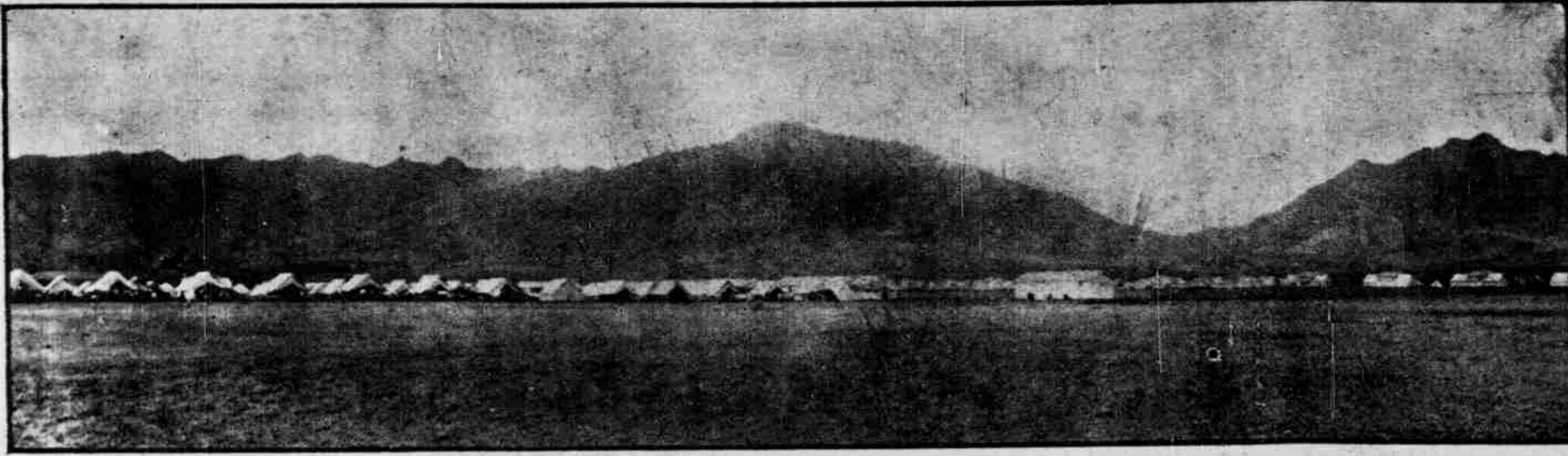
GENERAL VIEW OF TENT QUARTERS OF FIFTH CAVALRY.
