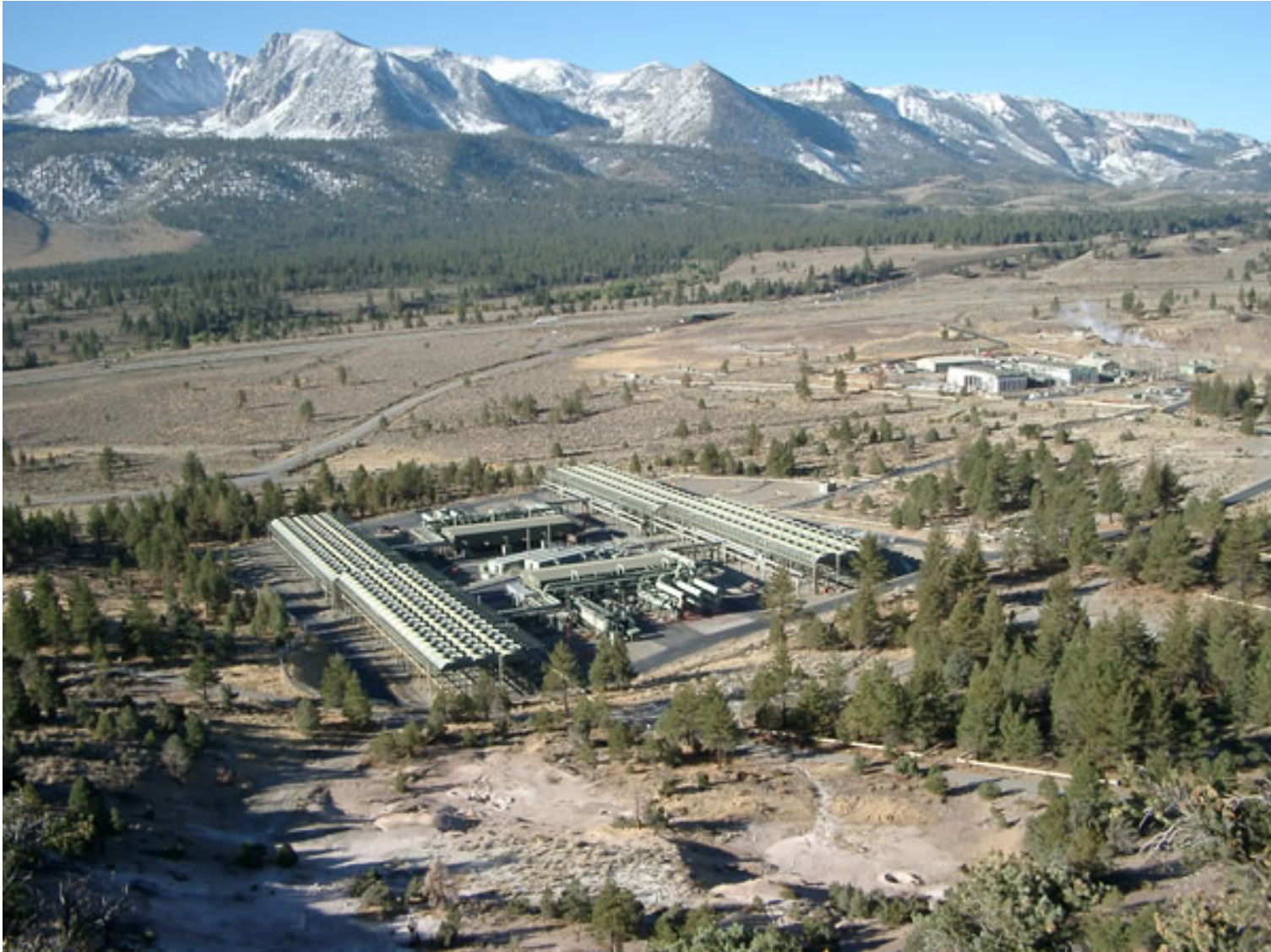
Figure 2.5: Aerial view of vegetation screen at Mammoth Pacific geothermal power plant (USDOI, 2014b).
