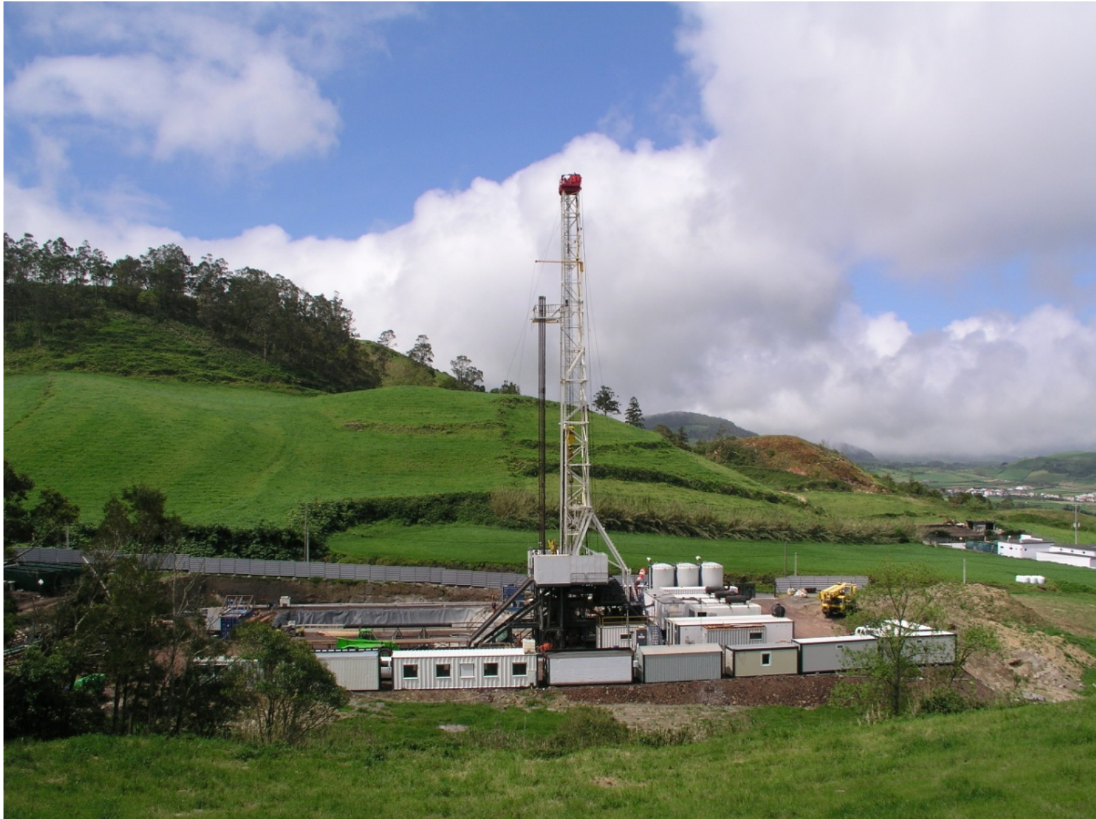
Figure 3.7: Drilling of a full diameter well.
