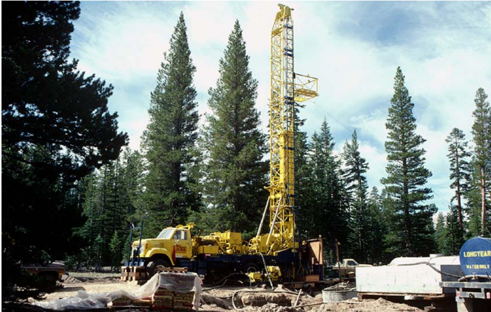
Figure 3.4: Drilling of a temperature gradient well.
