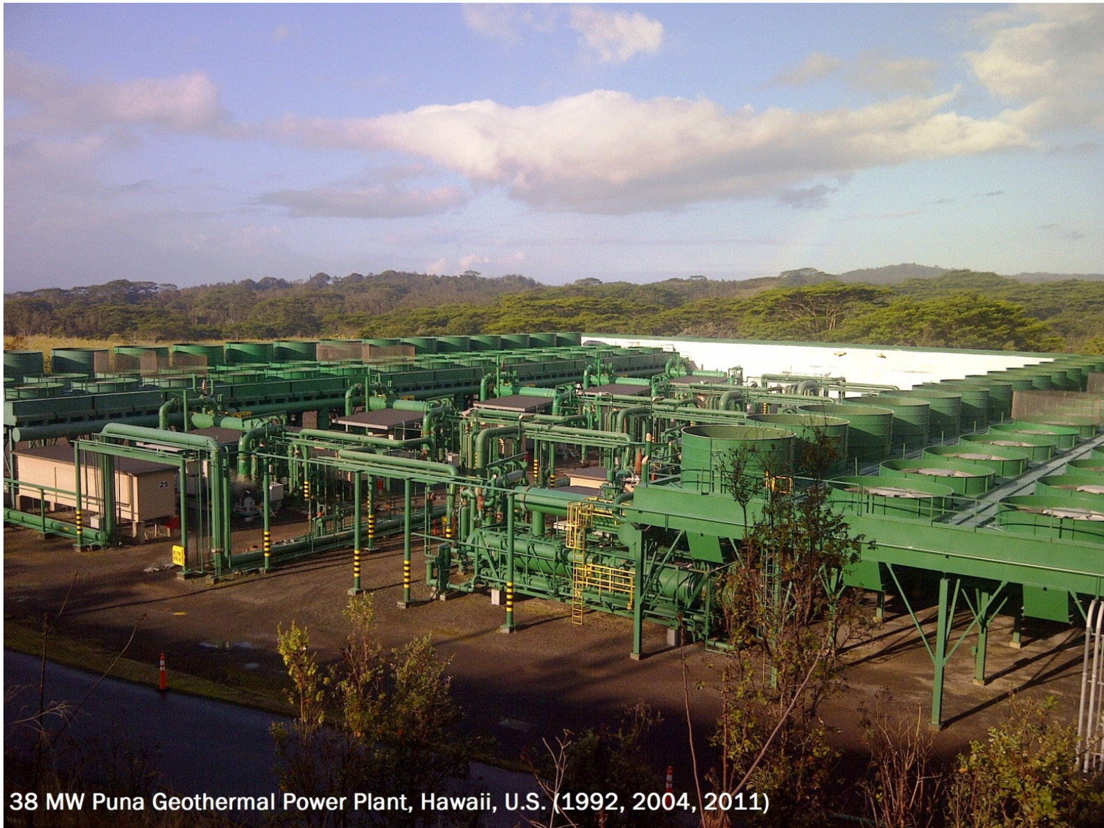
Figure 2.6: Air-cooled binary geothermal power plant at Puna (Photo courtesy of Ormat Technologies, Inc.).
