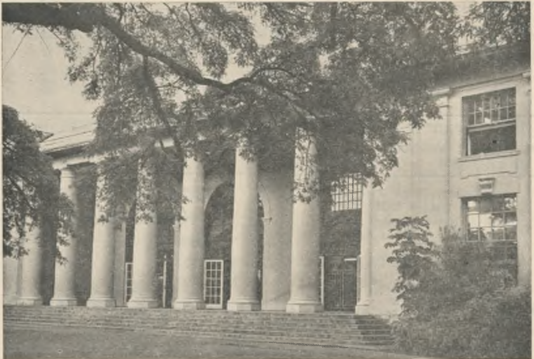
Among thousands of bound volumes, patrons of the central Library of Hawaii find intellectual treasures. Located ewa of Honolulu Hale (City Hall), the library includes also departments of music and art, and a Hawaiian and Pacific room. (Raymond C. Lum photo)
