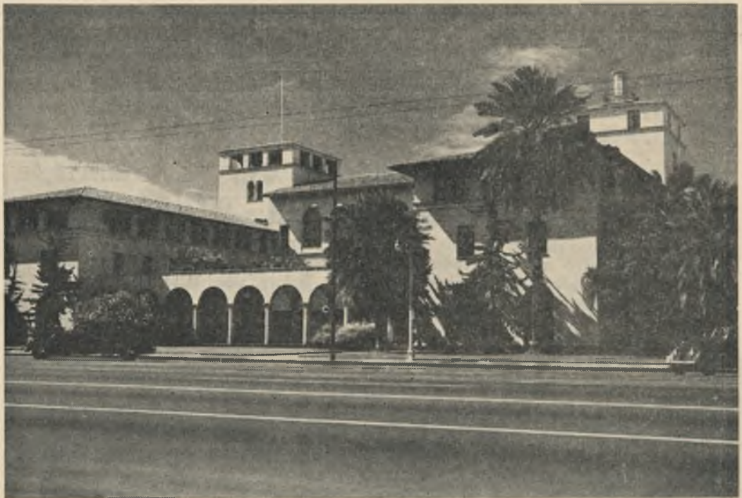
Across from the historic Iolani palace, the U.S. Government building houses the offices of the post office, public health service, weather bureau, and various othe federal agencies. (Raymond C. Lum photo) 富有歷史性意與蘭尼宮之對面，為中央政府機關大廈，內有郵政局，衛生局，氣象所，及其他中央機關代表辦事處。(林康熙攝影)
