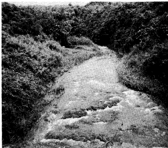
Figure 12 Waikomo Stream - View looking upstream from the new Poipu Road culvert.
