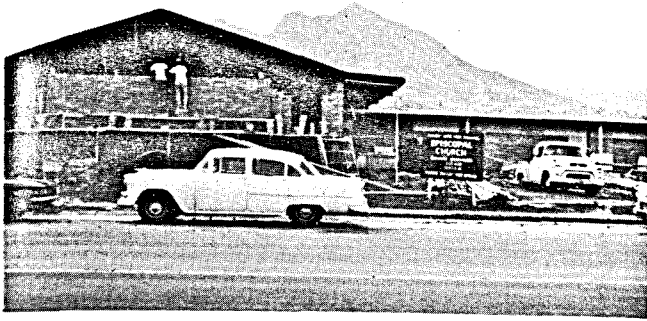
Emmanuel Church, Enchanted Lake—new parish hall and classrooms
