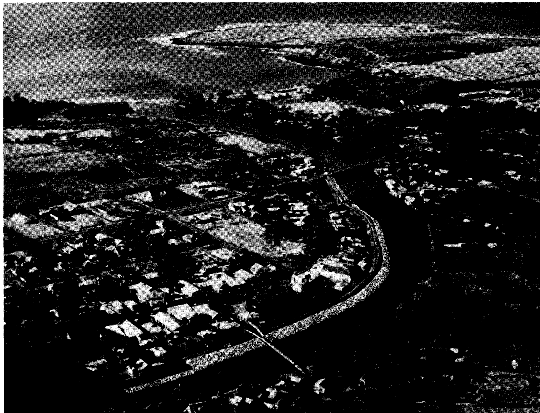
14. WORK ON THE LEFT BANK OF HANAPEPE RIVER, KAUAI, WAS COMPLETED IN 1959.
