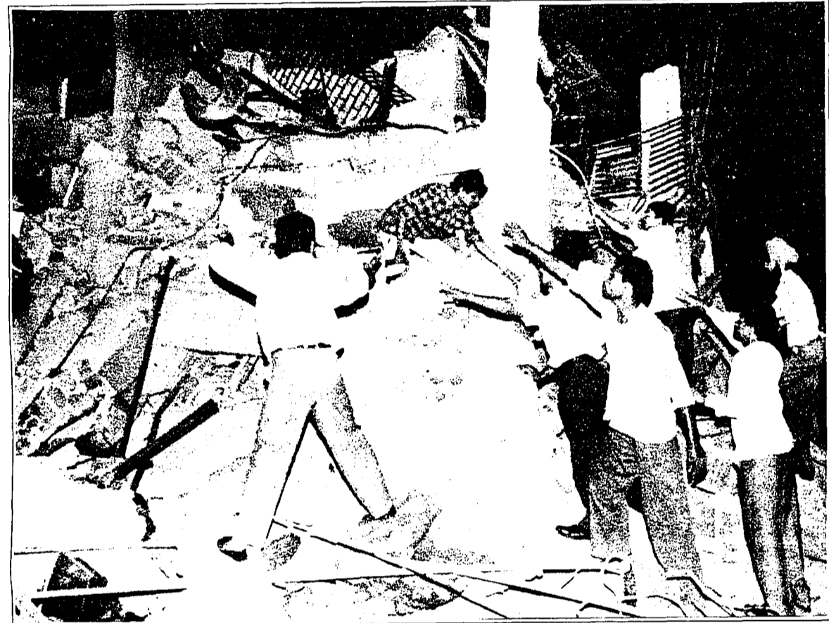
Residents from neighboring buildings offer their help in the rescue of people caught in the debris of a five-story building which collapsed in Bombay, India. Rescue workers continued to search for survivors Friday through the rubble of the collapsed building. At least 10 have died and 10 were injured in the accident. AP
