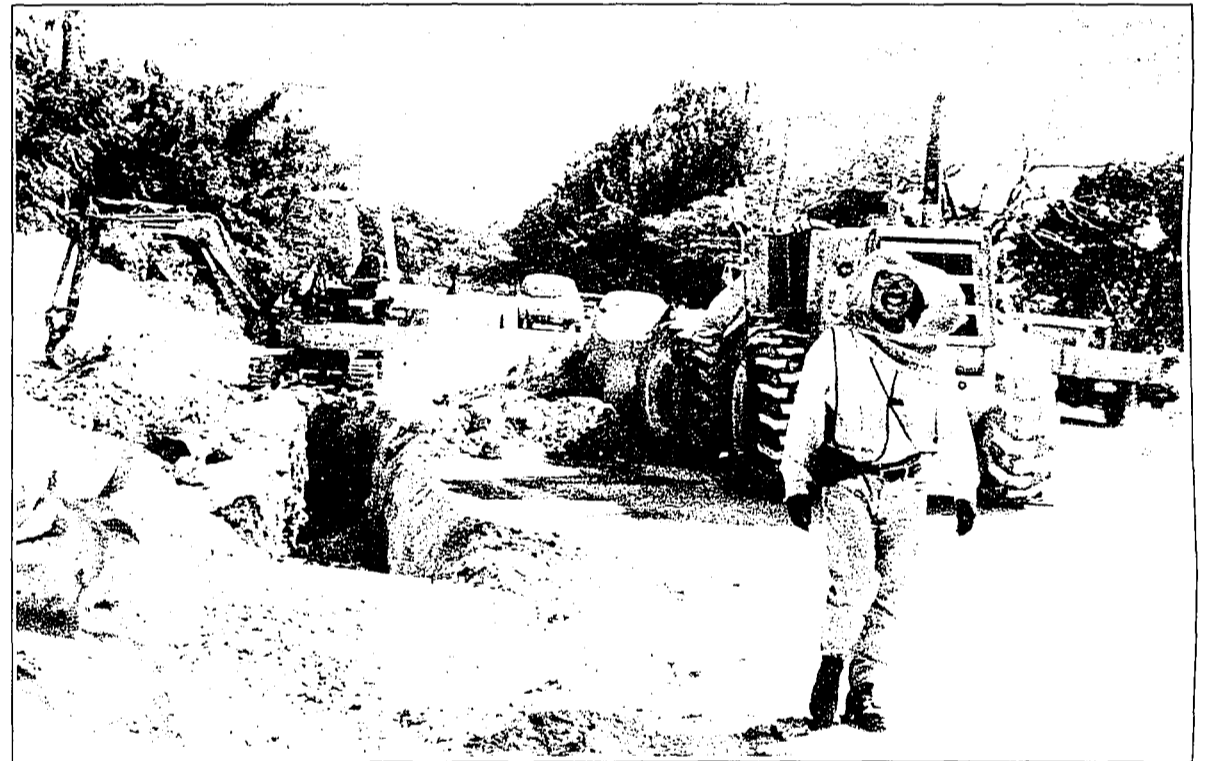
A heavy equipment operator walks away as a co-worker takes his turn in topping with soil a newly installed CUC water line along Beach Road near China House Restaurant in Garapan yesterday. A fire hydrant has been put up also in the area.
