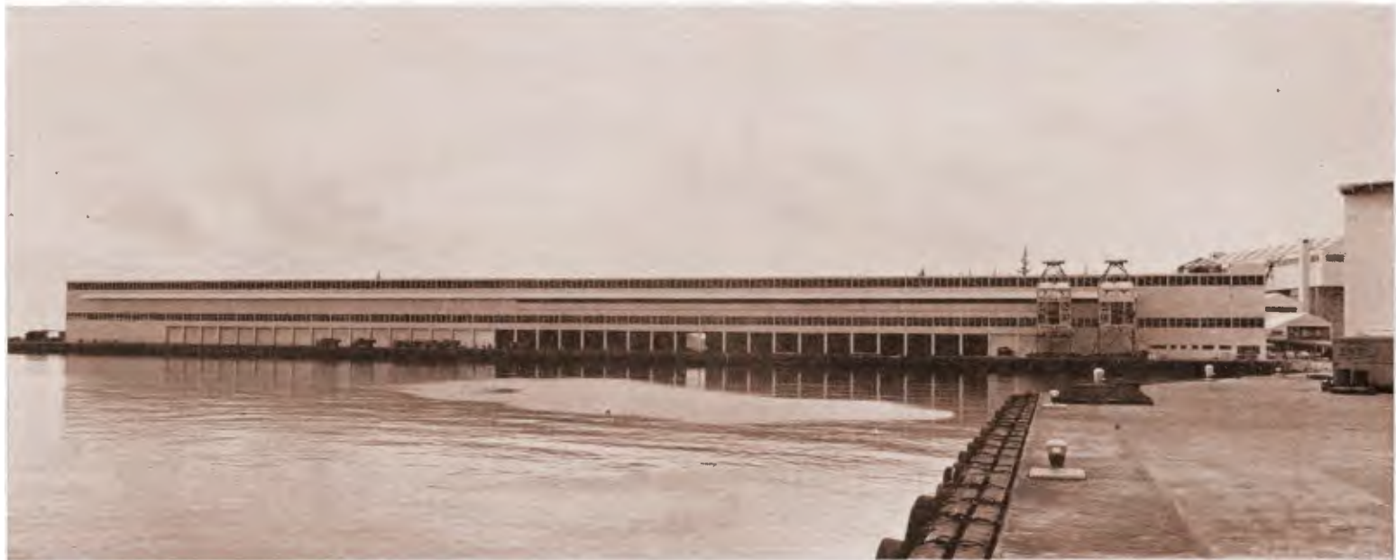
Pier 1 Hilo' after completion of reconstruction to replace shed destroyed by tidal wave of April 1, 1946. Shed is 1,040 feet long by 145 feet wide. Berthing face of concrete apron 1,172 feet.
