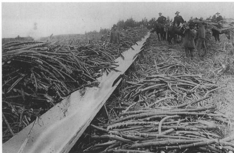
FIG. 2. Several plantations during this era used flumes as water transportation systems to get cane to the mill. Here workers are loading cane from ox carts onto the flumes. (Hawaiian Historical Society)
