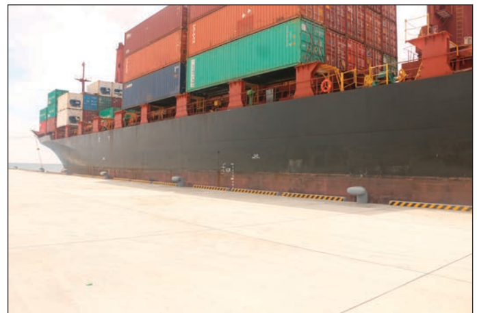
SIPA's new $190 million wharf was officially opened on 10th October, 2016. This Japan funded project will boost Solomon Islands international trade in goods. [Photo supplied by Solomon Star]
