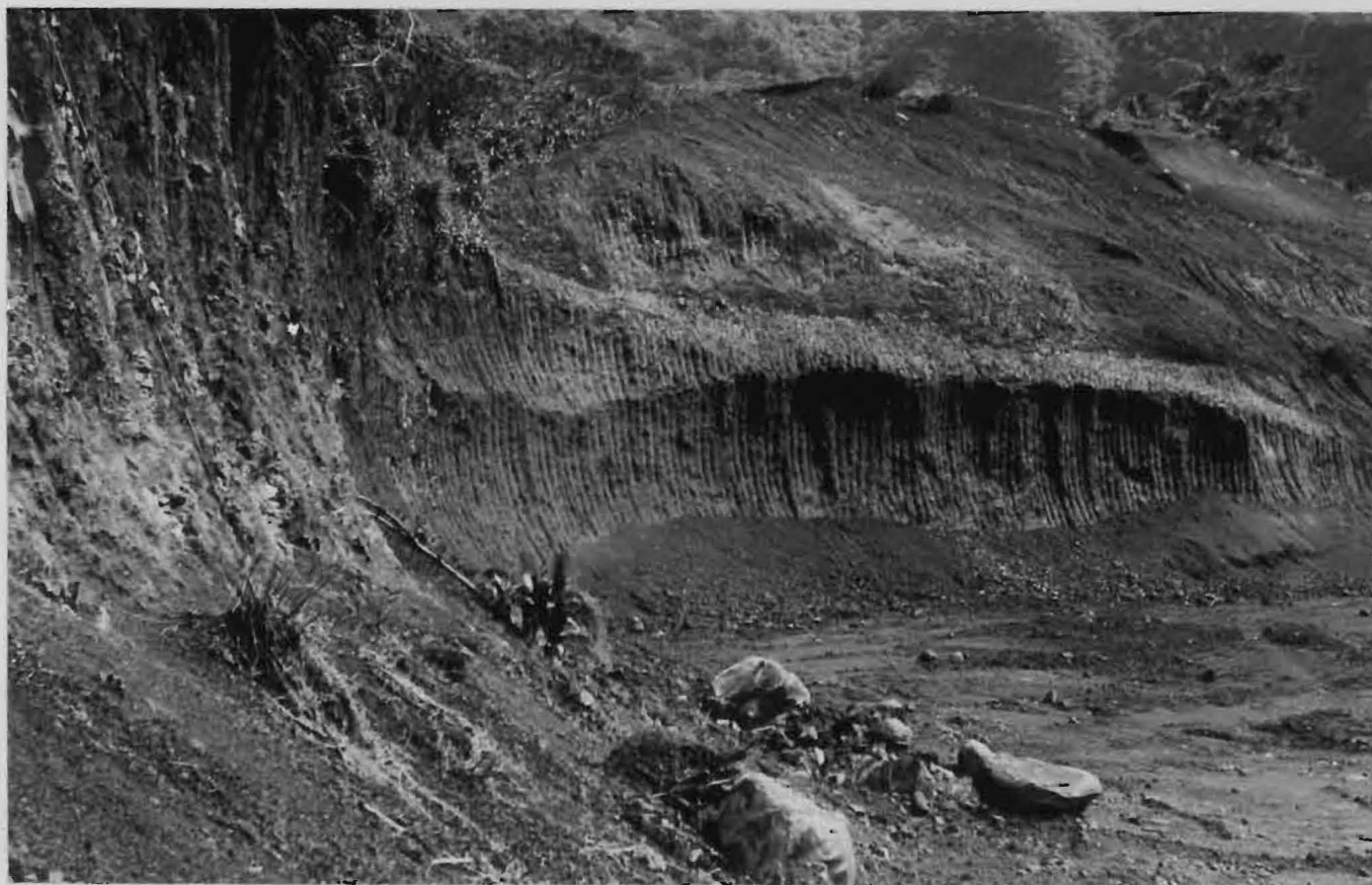
Figure 25 - View of borrow pit in old alluvium at No. 4 Dam. The floor of the pit and the walls marked by steam shovel teeth, are in weathered, mottled, old alluvium ranging from sand size to boulders 4 and 5 feet across. A few boulders from the upper part may be hard, but the general character of this old gravel is shown by implication in the steam shovel markings. This is typical of the sedimentary formations which make up the cap rock. (Negative No. 12006)
