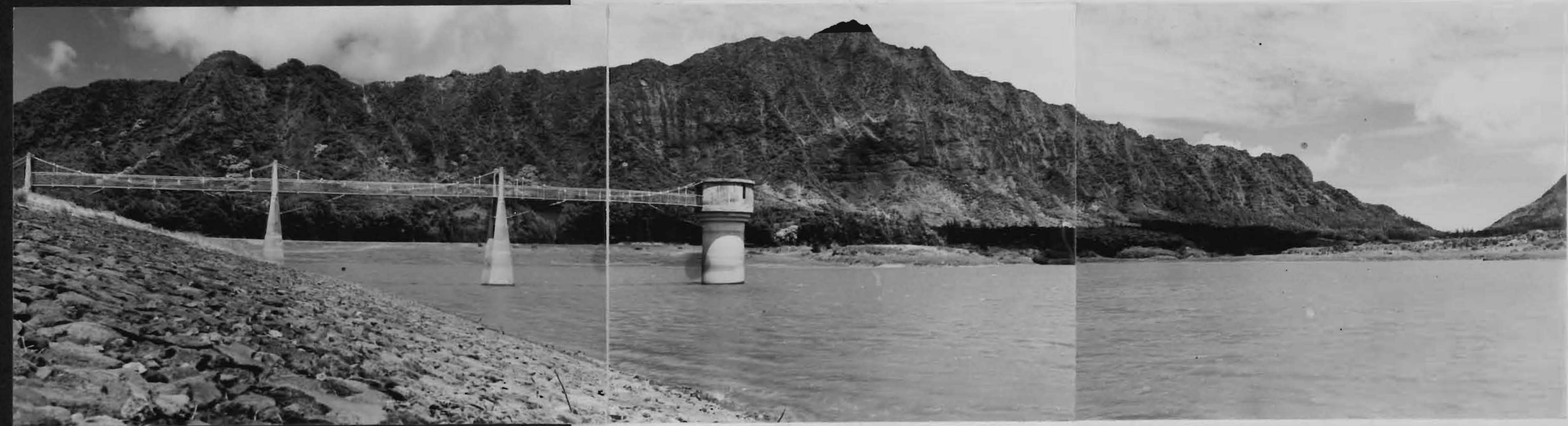
Figure 56 - Panorama from upstream face of Reservoir No. 4 to Lanihuli and west wall of Nuuanu Valley, showing gage tower and access bridge. (Negatives 13783-4-5, September 13, 1939)
