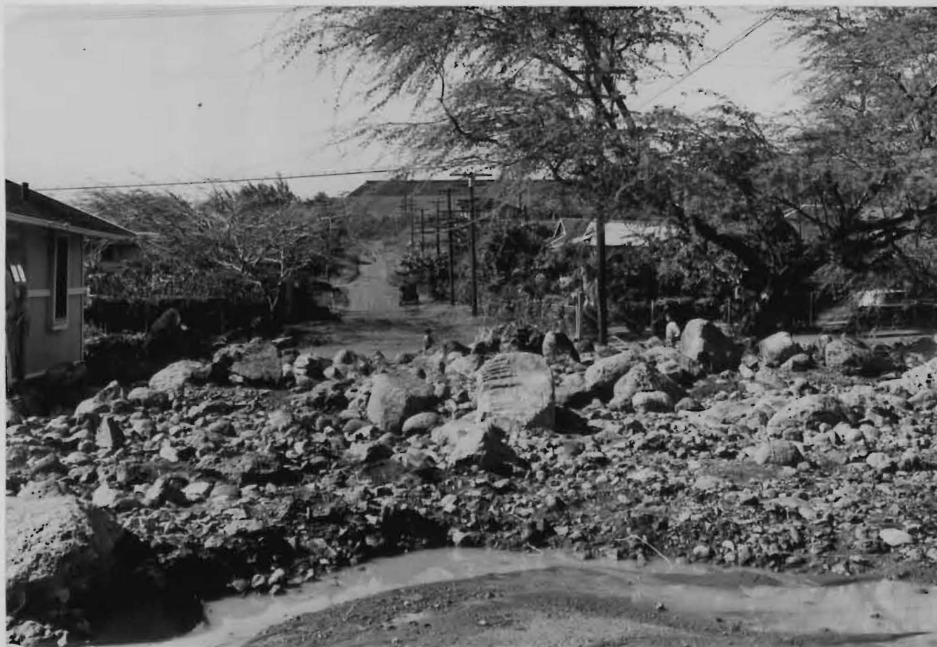
Figure 49 - Boulder gravel deposited on Konia Street east of Houghtailing Street during flood of February 27, 1935. View is looking northwest along Konia toward Houghtailing. The flood flow of Niuhelawai with a drainage basin approximating 300 acres exceeded the capacity of a culvert passing diagonally under both streets at the intersection, and the channel and culvert became blocked, passing the flood over Konia Street and forming a deposit of several hundred cubic yards, with boulders up to 7 by 4.5 by 2 feet and a total of 11 boulders measured at over 1 ton (12 cubic feet) each. (Negative No. 12416)
