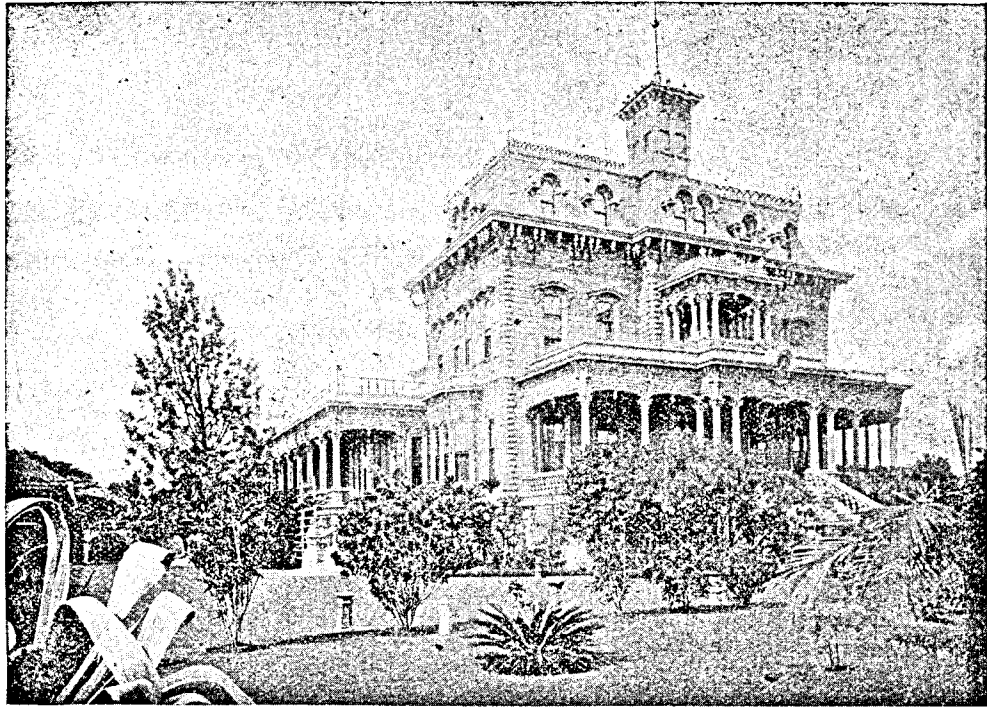
NEW HIGH SCHOOL BUILDING, EMMA STREET, HONOLULU.
