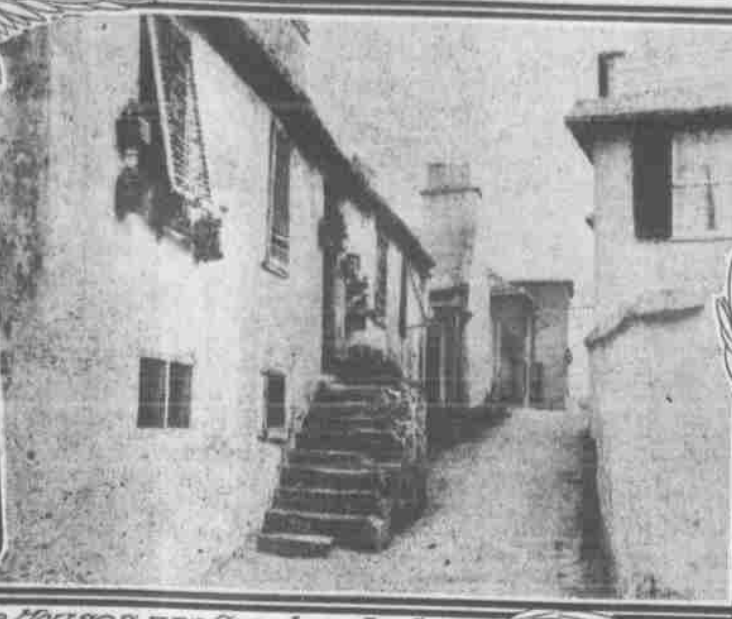
The houses are constructed of coral
