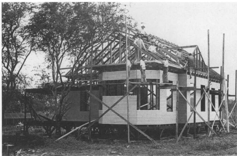
FIG. 4. Carpentry Shop students building a school cottage 1902–1903, Kamehameha School for Boys. (left to right, first row) Charles Brickwood Lyman (1904), Kaumu Hanchett (1904); (second row) Mr. Ira Eskew, Instructor, David Desha (1905), Arthur Arnold (1905); (third row) Stephen Desha (1903). Kamehameha Schools Photo Archives. Luryier Diamond, photo archivist.
