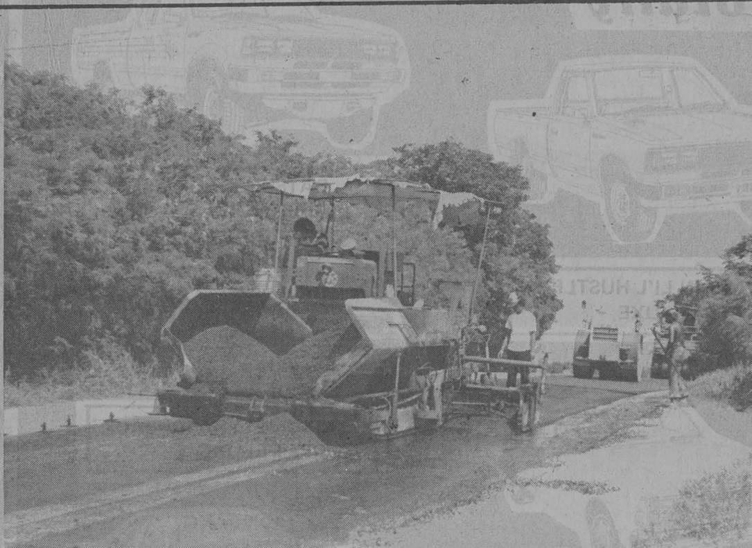
OLD SMOOTHIE — Maeda-Pacific construction workers laid down the first of two asphalt coats on Wallace Highway this week. Drivers had been complaining about the numerous potholes caused by the washing away of coral base.
