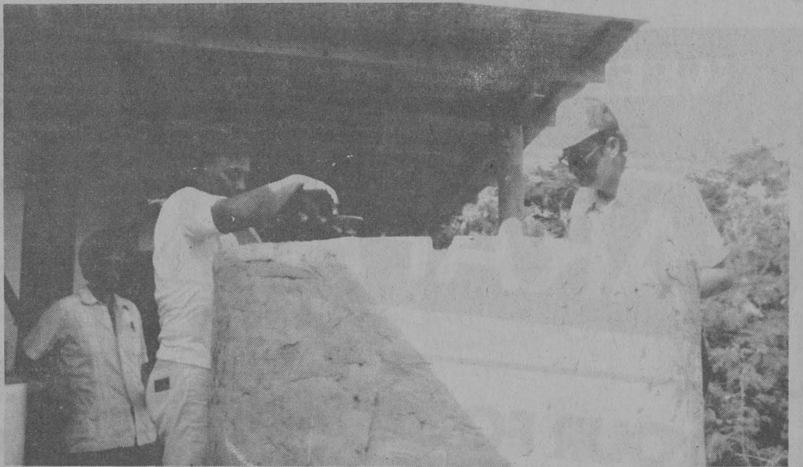
FOR CLEAN WATER — Final touches are put on a ferro-cement water tank built during a recent workshop for Peace Corps volunteers (Photo by N. Siren)
