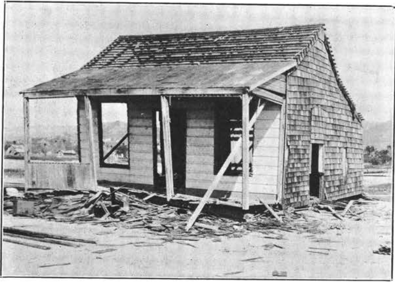
Illustrating the destructive work of the drywood inhabiting termites in parts of Honolulu.
