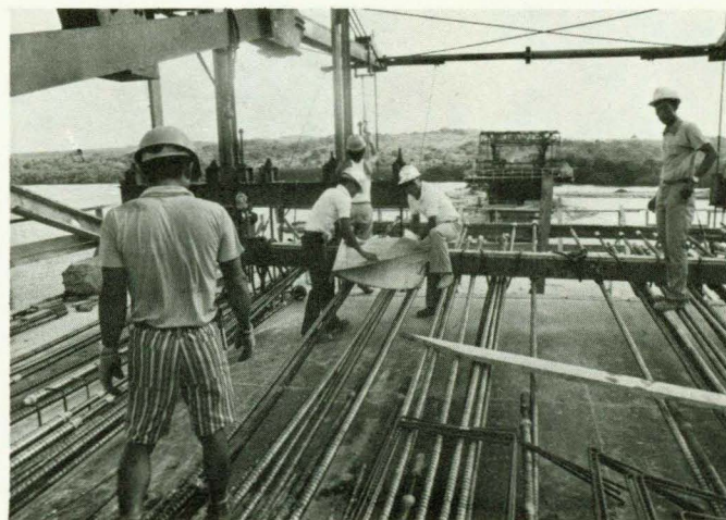
Laying out the reinforcement rods required highly professional skills and had to be done according to the bridge's blueprint.
