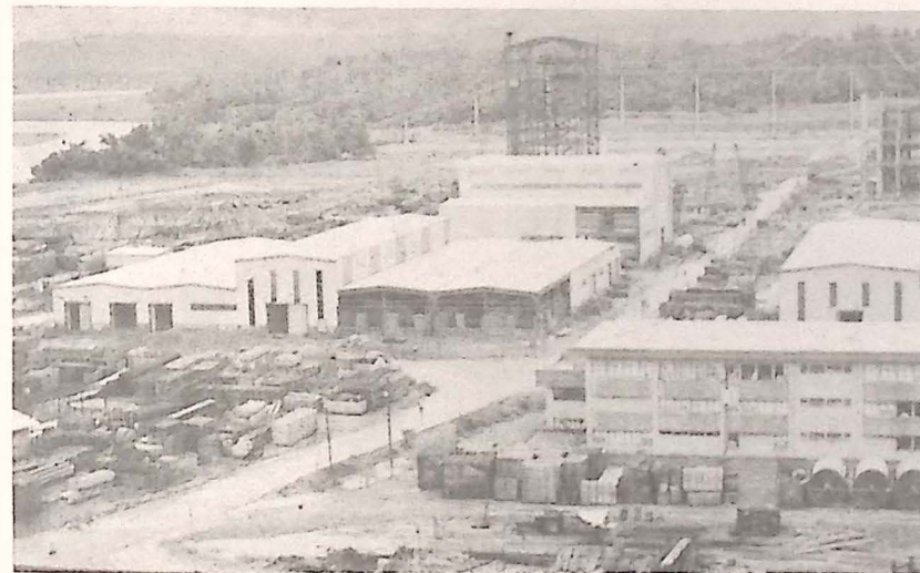
CRC's pulp mill complex
