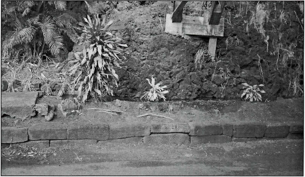
Figure 2. Section of Kikīaola (the Menehune Ditch).
