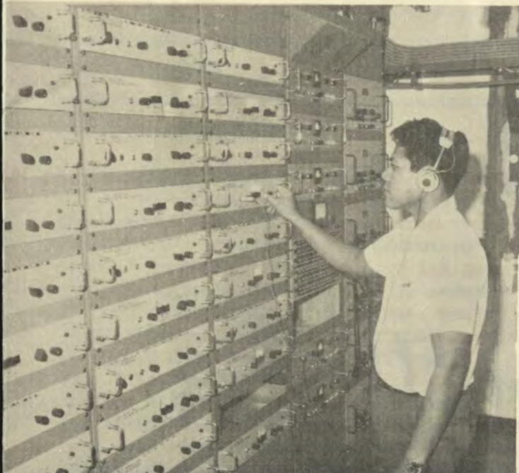
Mr. Miguel Sablan of EMD Kagman Relay/Control Station, tuning the receivers
