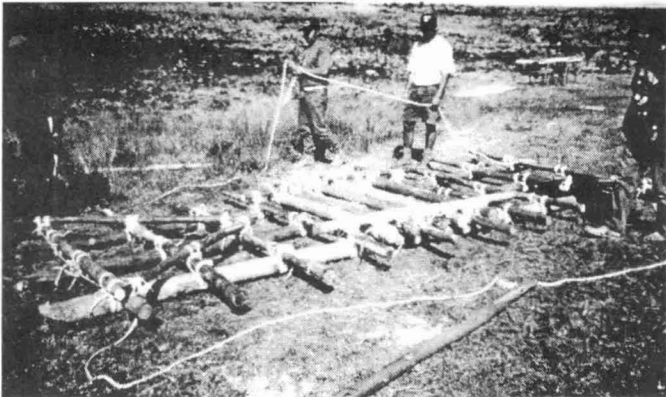
The V. R. Lee sled under construction.
