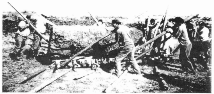
The V. R. Lee sled loaded and being levered 180°.
