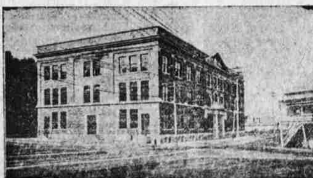
GENERAL STOREHOUSE, JUST COMPLETED, THE LARGEST BUILDING IN THE PORTSMOUTH NAVY YARD, IN WHICH THE PEACE ENVOYS WILL CONFER.
