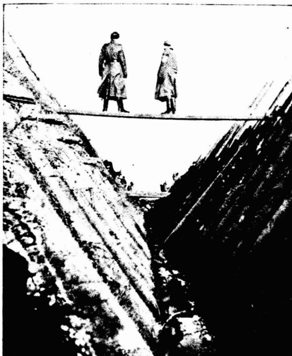
All along the German frontiers hundreds of thousands of Germans are busy building antitank trenches such as this one
