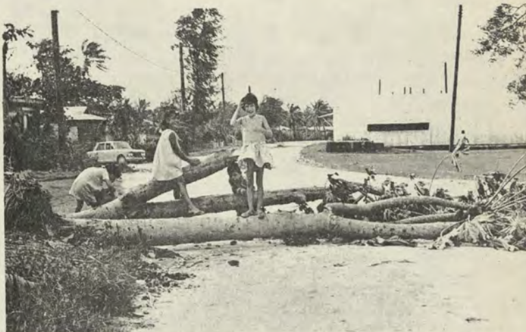
Children play on fallen tree in Chalan Kanoa, behind the elementary school. Although most damage in Saipan was confined to fallen debris on roadways, a few houses, like the one below in San Vicente Village, suffered considerable damage.
