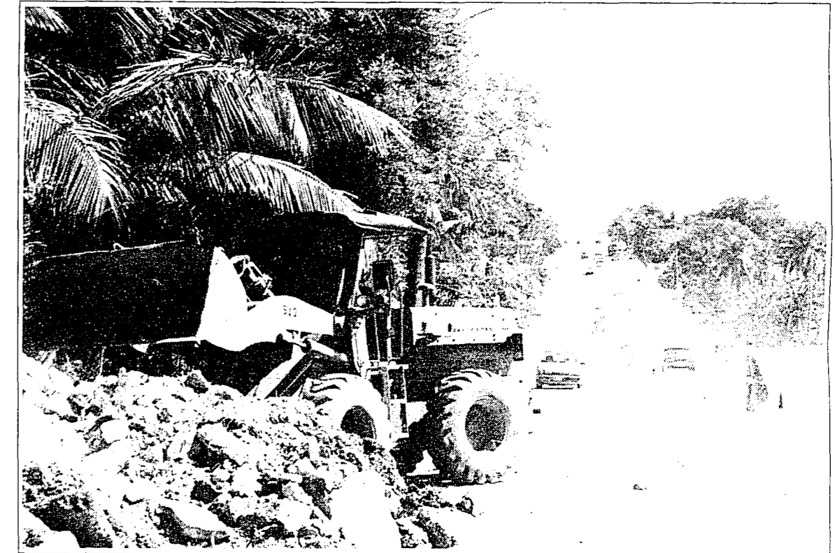
COUNTDOWN. Workers rush the completion of the 2-kilometer portion of the Monsignor Guerrero road. Public Works Secretary Edward DL Guerrero said the project, planned to be done by Dec. last year, will be completed March this year. Photo by Jojo Dass
