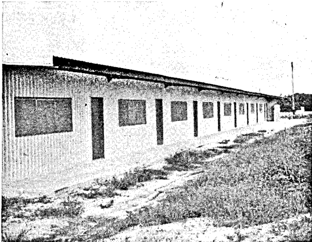
New classroom building at St. John's the Divine, Agana, Guam, built to replace the one destroyed by the typhoon last year.
