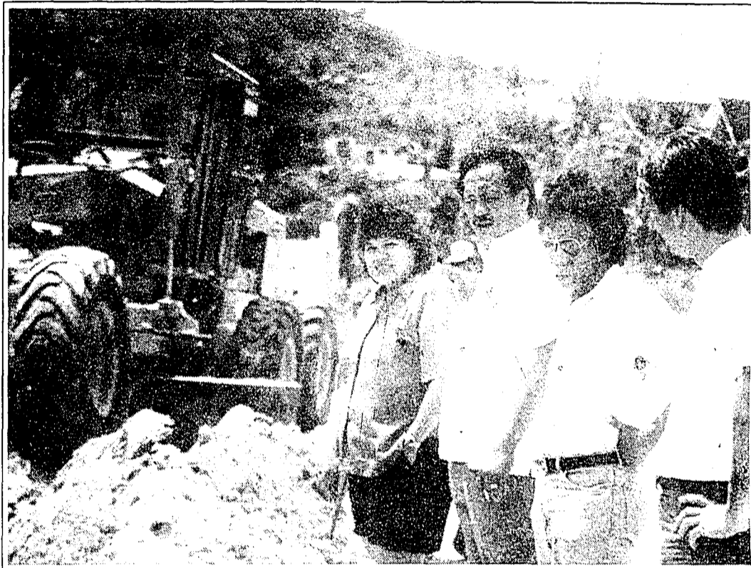
DPW Director Elizabeth Balajadia supervises Road paving project of Dandan Road with Public Works Inspector from Guam.
