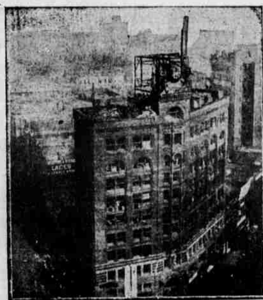
THE CHRONICLE BUILDING AFTER THE RECENT FIRE.
