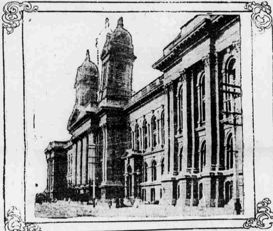
SAN FRANCISCO'S CITY HALL, WHICH COLLAPSED AT THE FIRST SHOCK.
