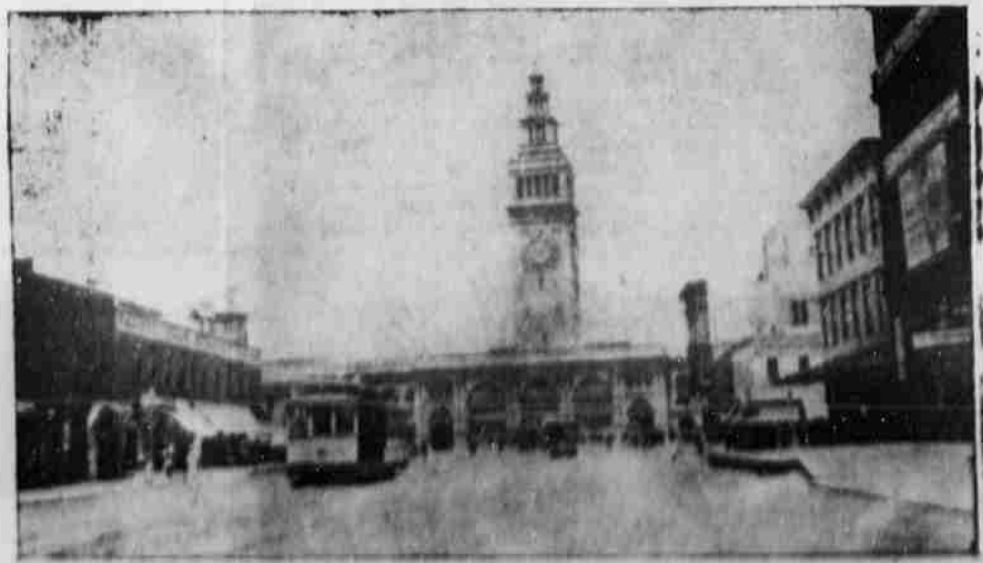
THE FERRY BUILDING, FOOT OF MARKET STREET.
