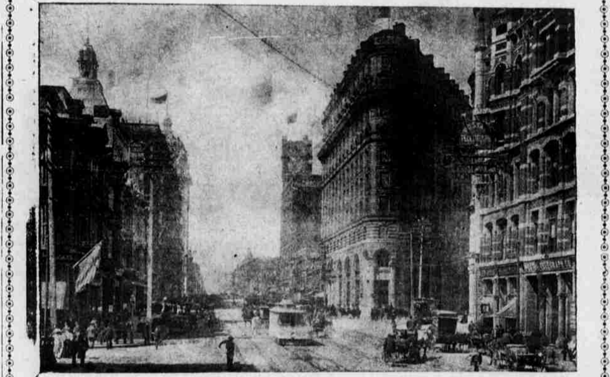
VIEW OF MARKET STREET—THE BUILDING AT THE RIGHT OF THE PICTURE, CONTAINING THE CABLE OFFICE, IS AMONG THE NUMBER BURNED.
