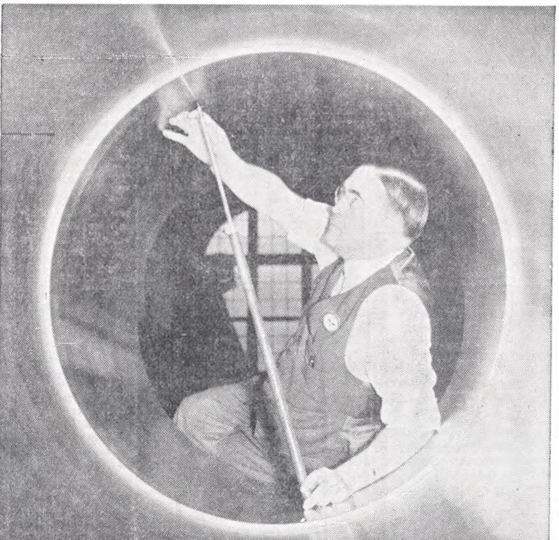
Imagine waking from a nightmare and having this big gun stare you in the face! A highly skilled inspector is shown checking the bore of the hoop of a big weapon in arsenal at Watervliet, New York. Note identification badge he wears.
