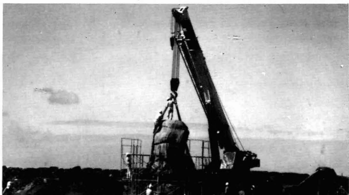
Reconstruction of Ahu Tongariki underway in 1993 using the crane donated by Tadano Corporation (photo by R. Morales).
