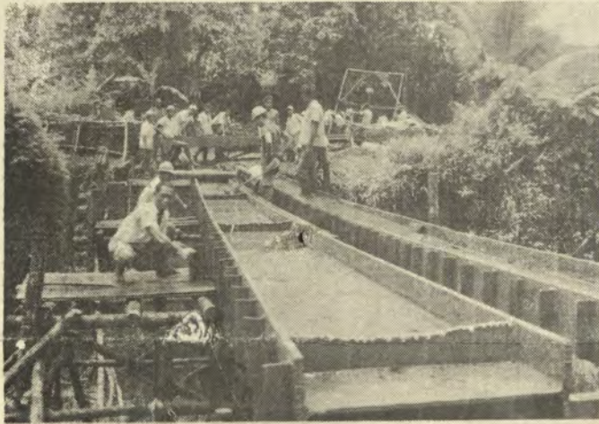
ROLLING THE BEAMS down the road and across river.
