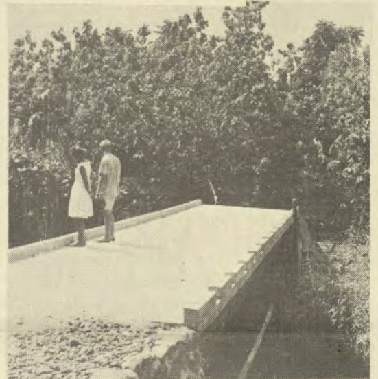
LEHDAU I BRIDGE serves pedestrians and vehicles.
