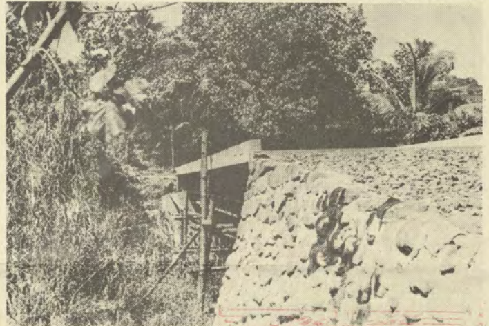
FIFTY CUBIC YARDS OF ROCK used in the approaches.
