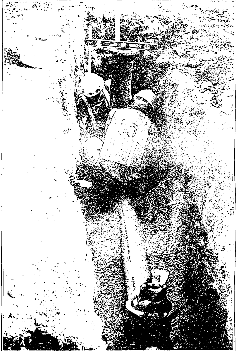
Workers from Sablan Construction arrange fittings for the huge PVC pipes they have installed underground. The work is part of CUC's waterline improvement project in front of the Cabrera Center in Chalan Laulau.
