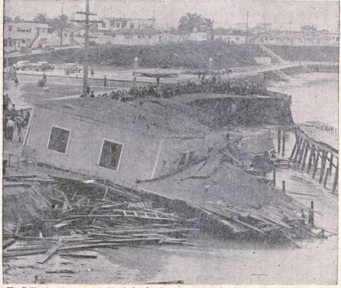
The California storm season, starting in Los Angeles area, got in its first destructive licks when wind-lashed waves battered coast at Ocean Beach and destroyed property, as shown. Hundreds of curious sightseers gathered to view wreckage.
