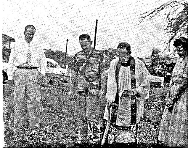
Groundbreaking service for St. Barnabas Church, Ewa Beach, Sunday, July 13, 1958, with the Rev. Arthur B. Ward, officiating.
