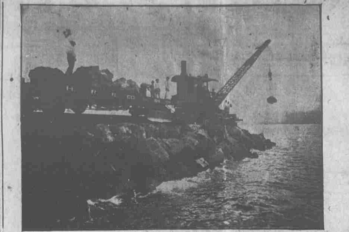
CONSTRUCTION WORK ON HILO BREAKWATER.
