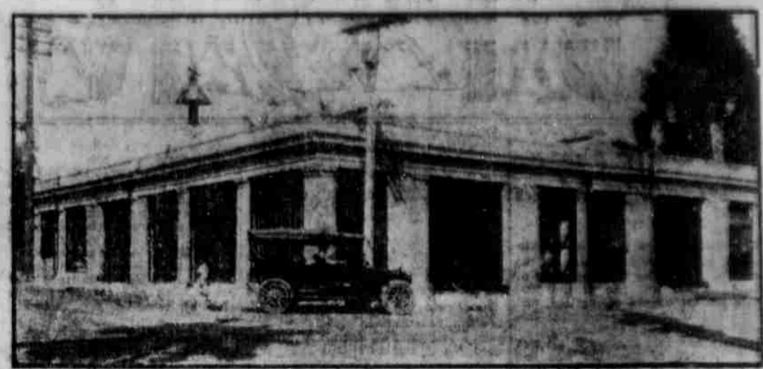
NEW HILO GARAGE. Showing how simple it is to combine art with utility in construction.
