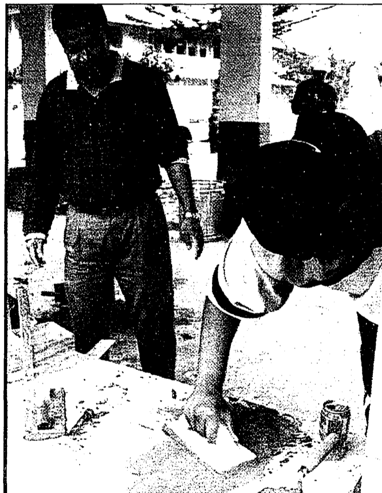
MHS Construction Instructor Joven Mallari assists a student in finishing work on a campus concrete bench. The students are constructing several benches along the school's entrance as part of a class project.
